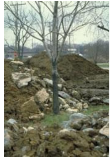
5. Soil and debris piled on the construction site can smother roots.
