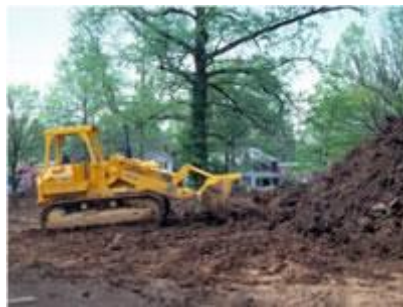
Figure 4. Heavy construction equipment compacts soil in the tree root zone.
