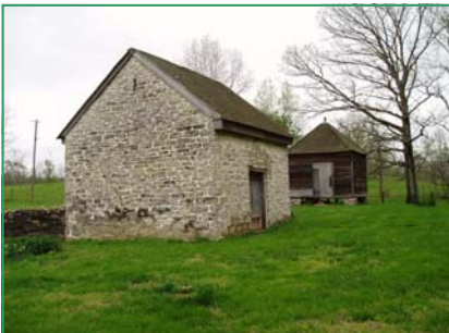
“This the smoke house or meat house on the Jullian Farm that is still mostly original. Outbuildings for the survey don’t need to be this nice or unique to qualify, simple board and batten or rough saw structures can qualify just as well.”
