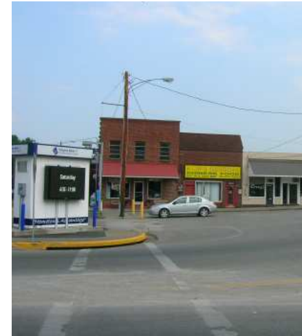
Crosswalks are minimally delineated and provide inaccessible transitions between sidewalk and roadway.
