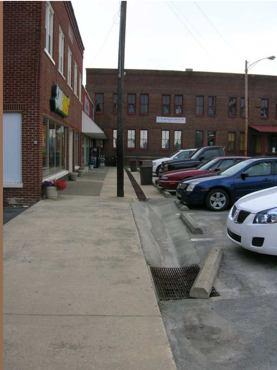
Existing Photo of Southeast Quadrant of Downtown Square
