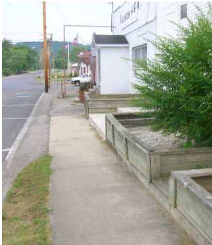
Narrow sidewalks on southern edge of Upper River Street present potential accessibility issues.
